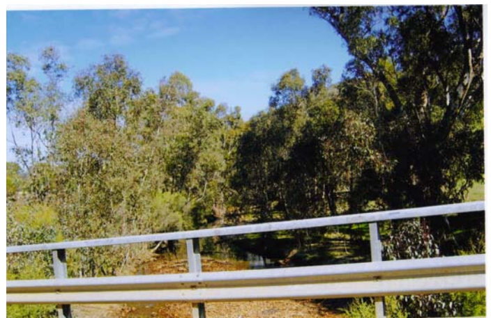
(R) - Tree growth from the new Jimperding Brook bridge
