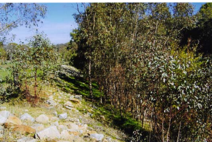
(L) - Section of 70 metre rock area to support Brook banks
